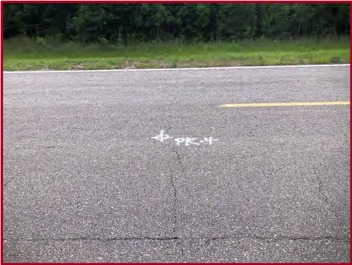
FIGURE D7: EXISTING CONDITIONS AT PAVEMENT CORE PK-4 (FACING EAST)
