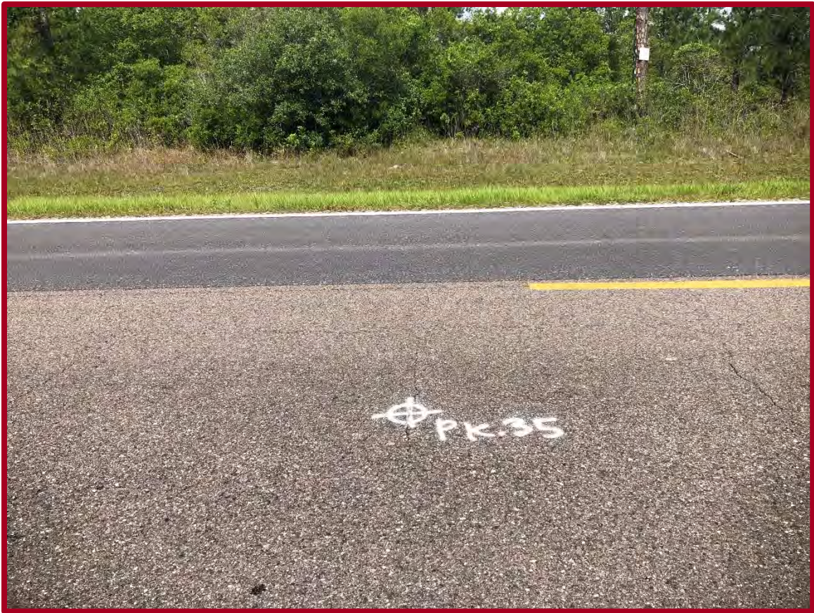
FIGURE D69: EXISTING CONDITIONS AT PAVEMENT CORE PK-35 (FACING WEST)
