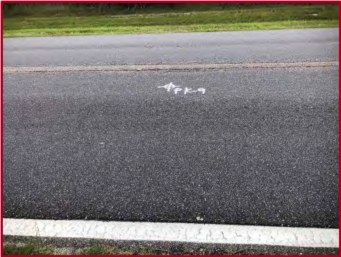
FIGURE D17: EXISTING CONDITIONS AT PAVEMENT CORE PK-9 (FACING WEST)
