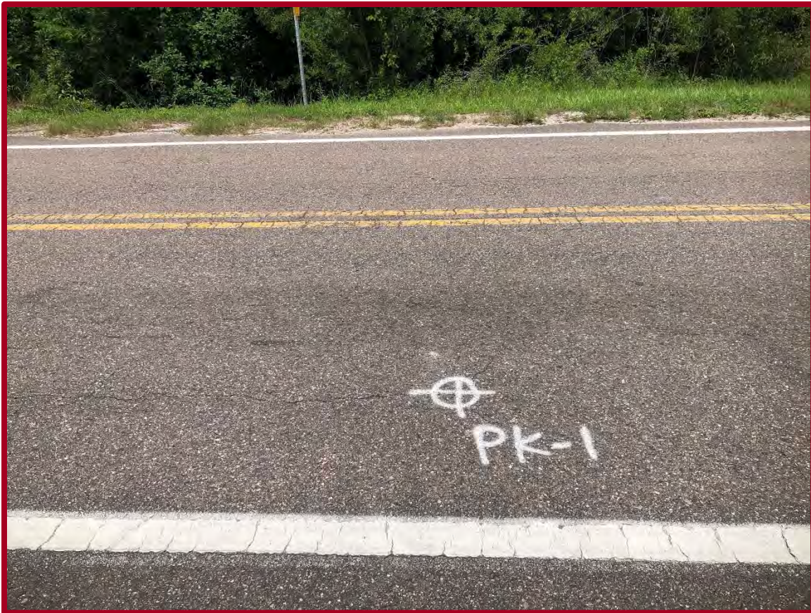
FIGURE D1: EXISTING CONDITIONS AT PAVEMENT CORE PK-1 (FACING WEST)
