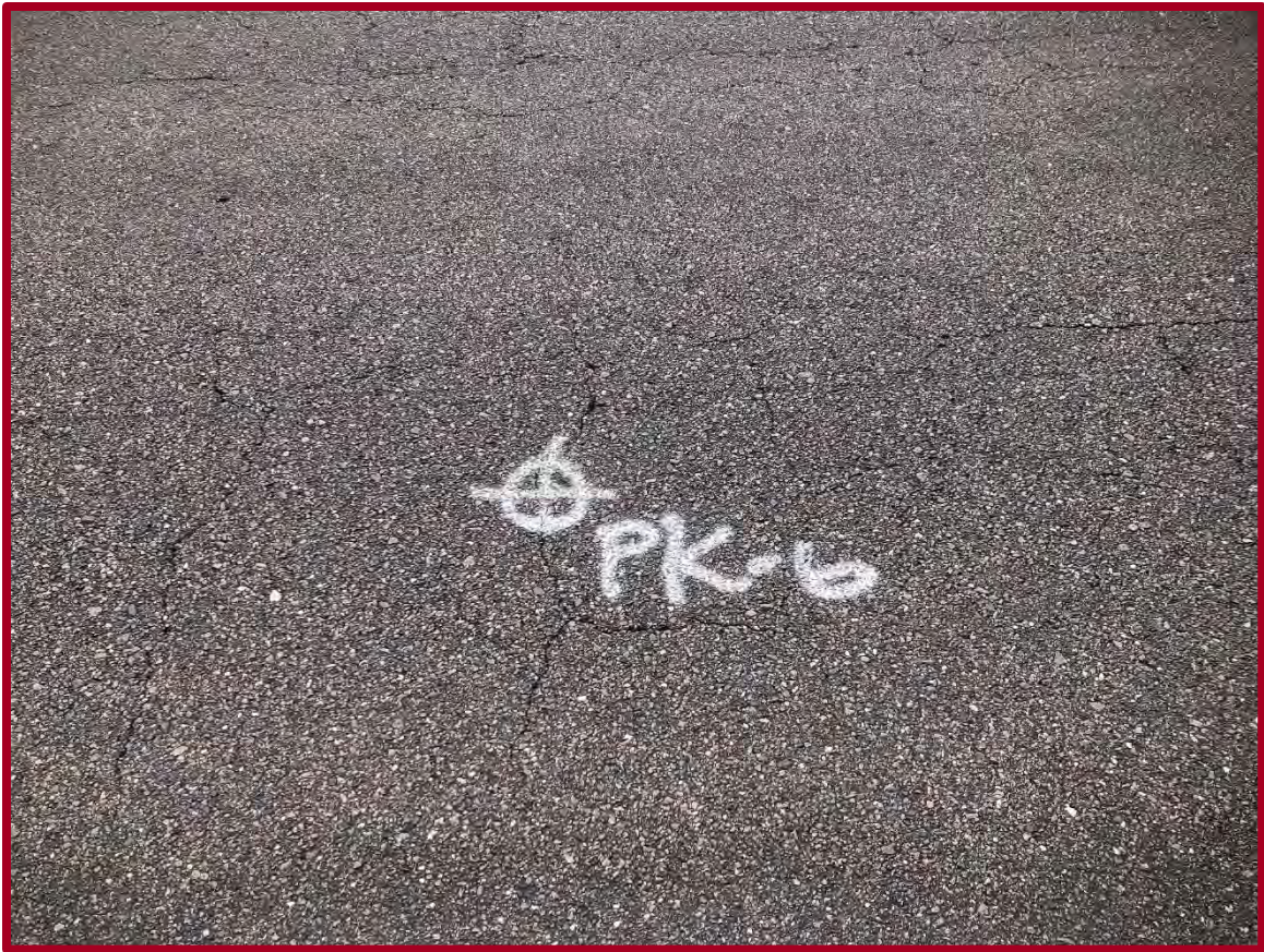
FIGURE D11: EXISTING CONDITIONS AT PAVEMENT CORE PK-6 (FACING EAST)
