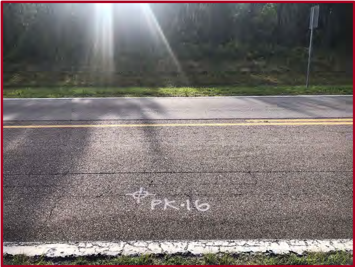
FIGURE D31: EXISTING CONDITIONS AT PAVEMENT CORE PK-16 (FACING EAST)
