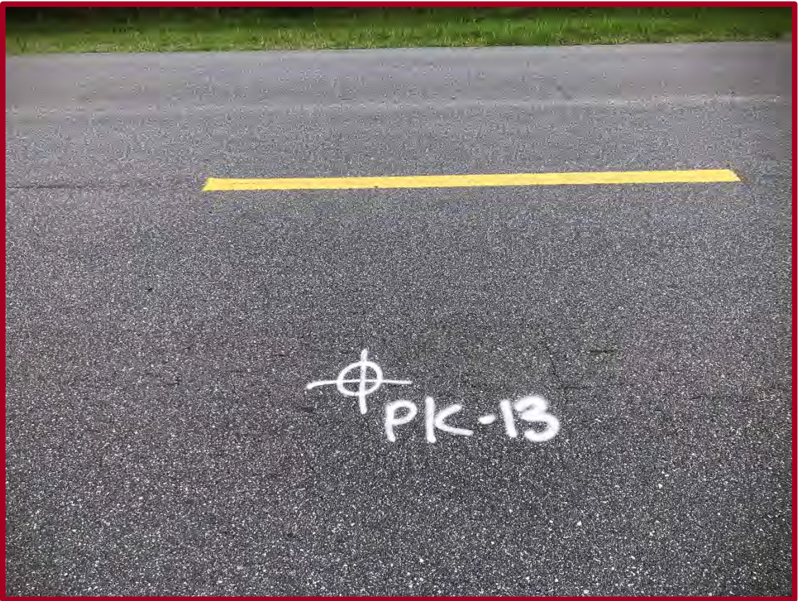
FIGURE D25: EXISTING CONDITIONS AT PAVEMENT CORE PK-13 (FACING WEST)
