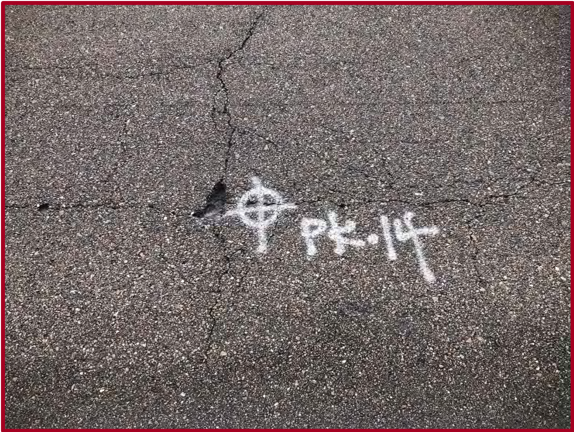
FIGURE D27: EXISTING CONDITIONS AT PAVEMENT CORE PK-14 (FACING EAST)
