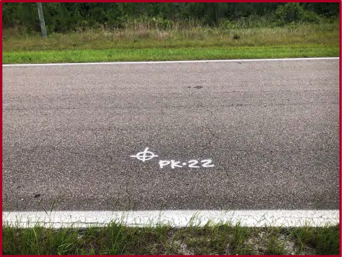
FIGURE D43: EXISTING CONDITIONS AT PAVEMENT CORE PK-22 (FACING EAST)
