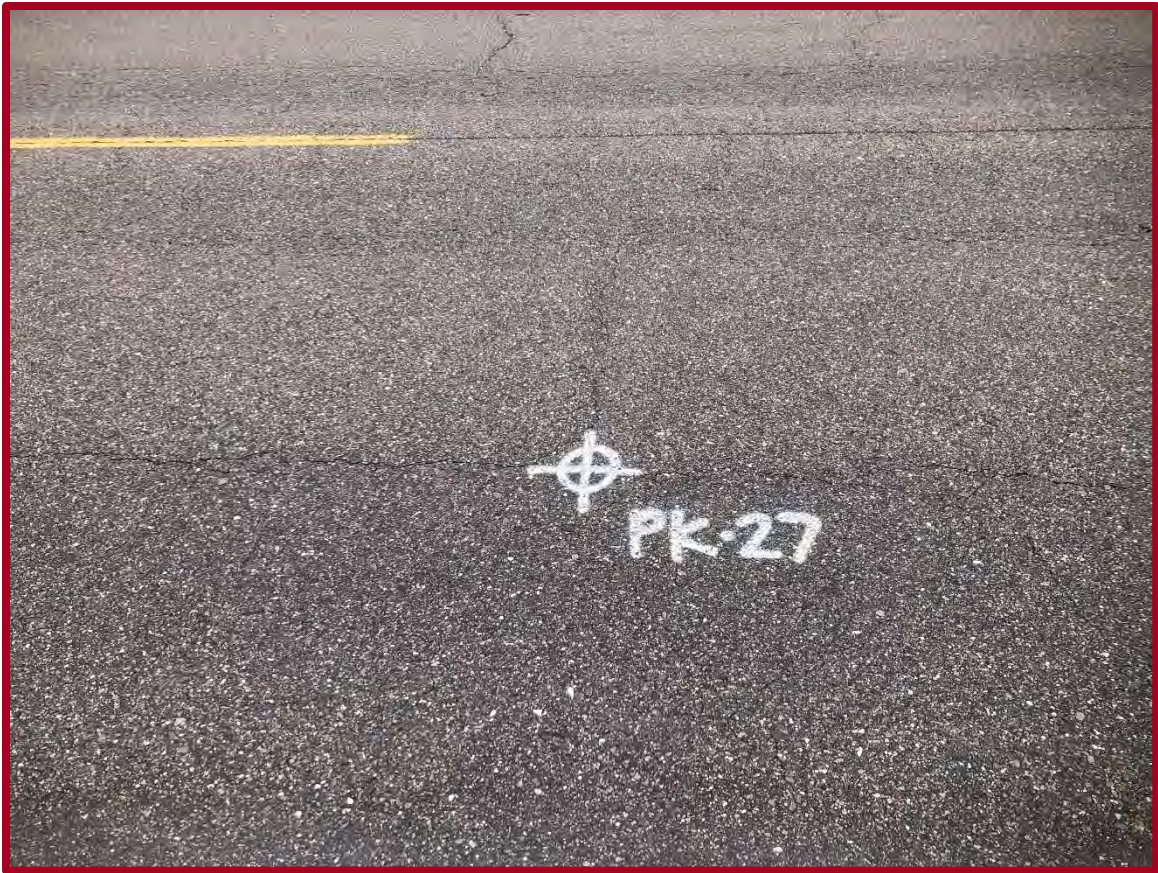
FIGURE D53: EXISTING CONDITIONS AT PAVEMENT CORE PK-27 (FACING WEST)
