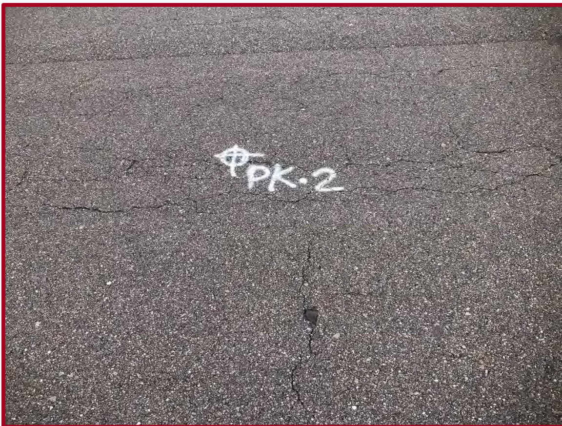
FIGURE D3: EXISTING CONDITIONS AT PAVEMENT CORE PK-2 (FACING EAST)
