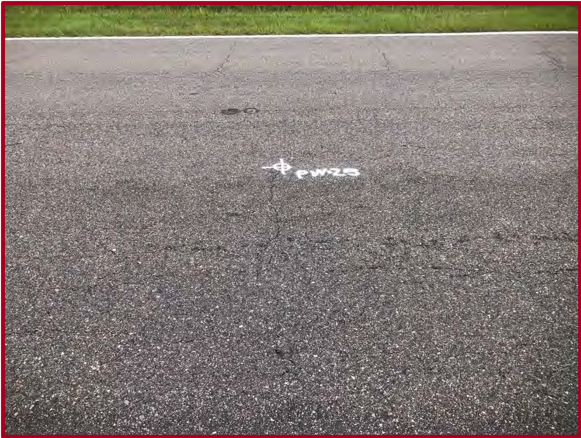
FIGURE D49: EXISTING CONDITIONS AT PAVEMENT CORE PK-25 (FACING WEST)
