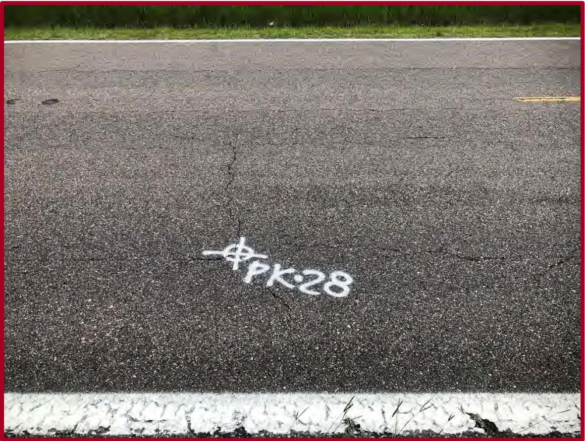
FIGURE D55: EXISTING CONDITIONS AT PAVEMENT CORE PK-28 (FACING EAST)
