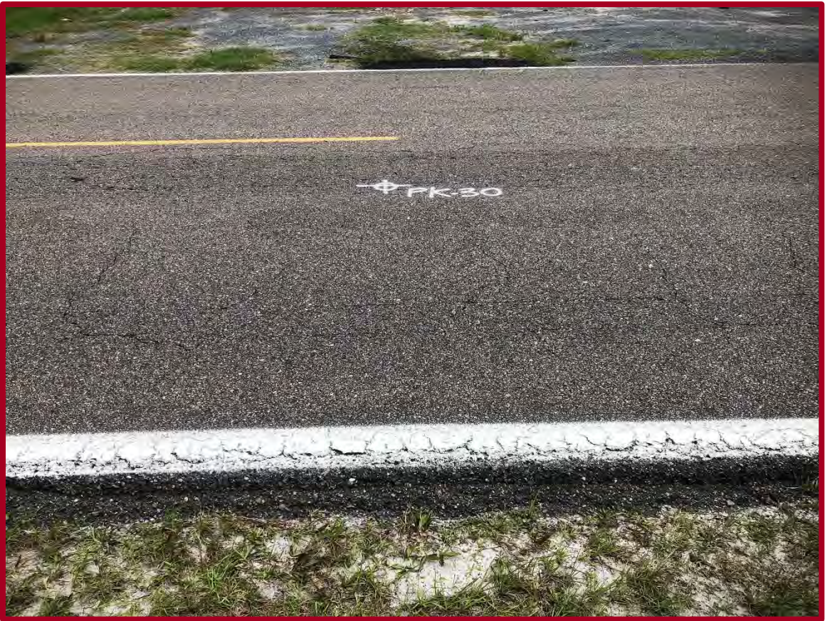
FIGURE D59: EXISTING CONDITIONS AT PAVEMENT CORE PK-30 (FACING EAST)
