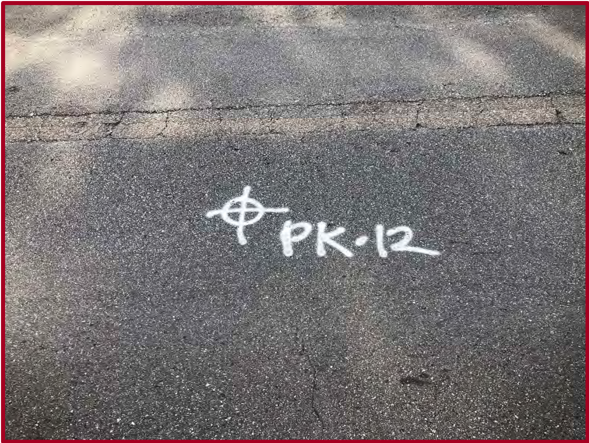
FIGURE D23: EXISTING CONDITIONS AT PAVEMENT CORE PK-12 (FACING EAST)
