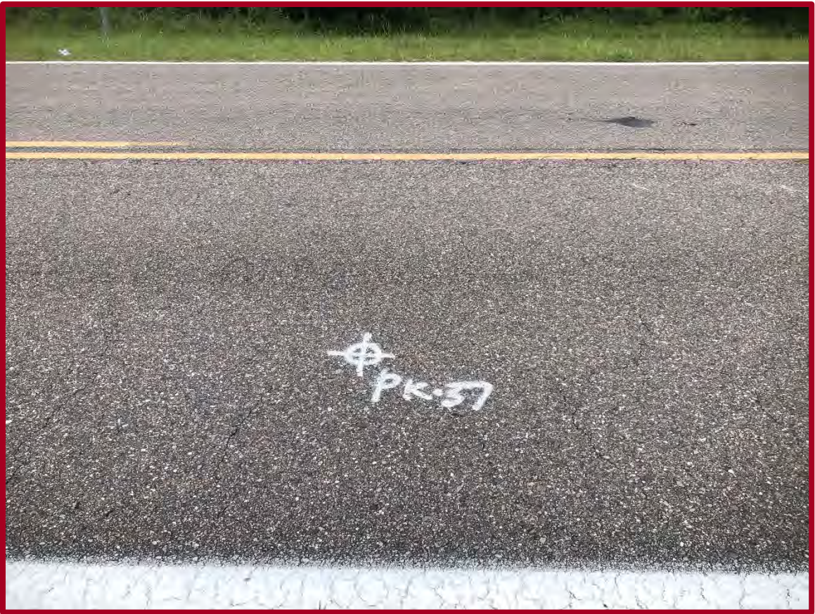
FIGURE D73: EXISTING CONDITIONS AT PAVEMENT CORE PK-37 (FACING WEST)
