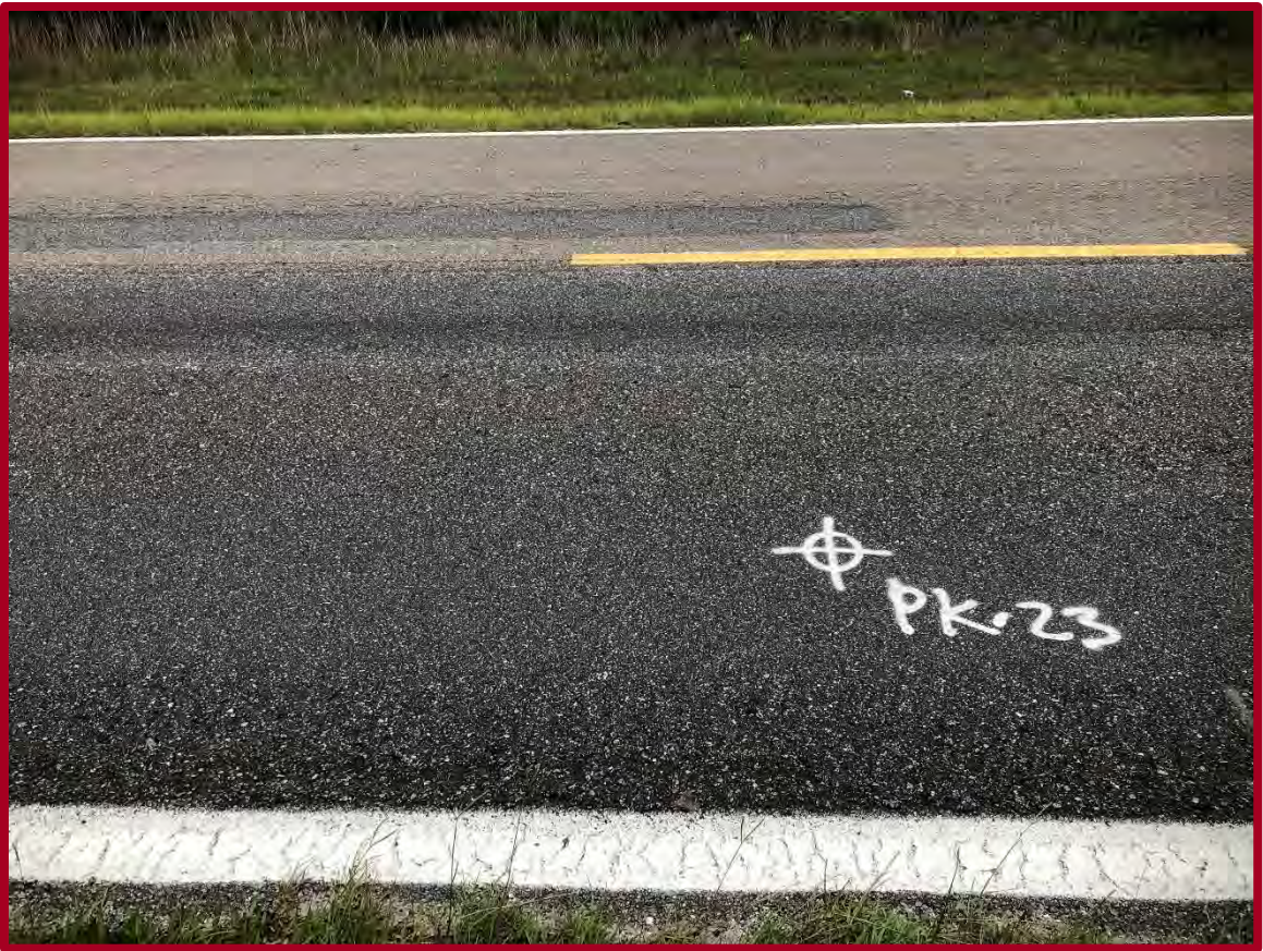
FIGURE D45: EXISTING CONDITIONS AT PAVEMENT CORE PK-23 (FACING WEST)
