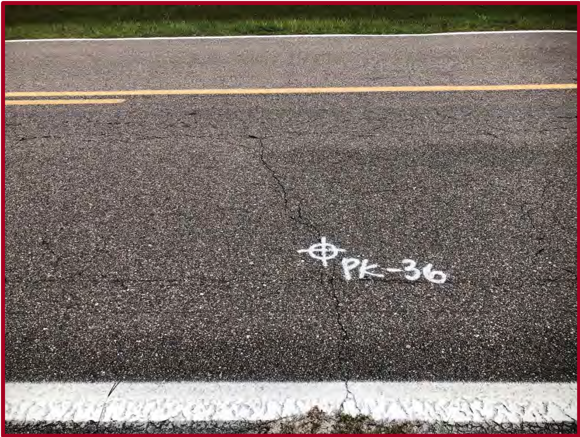
FIGURE D71: EXISTING CONDITIONS AT PAVEMENT CORE PK-36 (FACING EAST)
