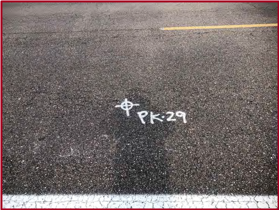
FIGURE D57: EXISTING CONDITIONS AT PAVEMENT CORE PK-29 (FACING WEST)
