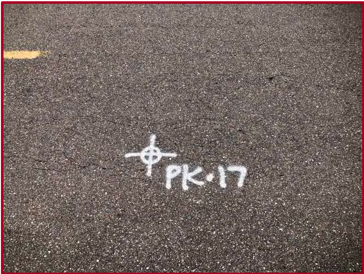
FIGURE D33: EXISTING CONDITIONS AT PAVEMENT CORE PK-17 (FACING WEST)
