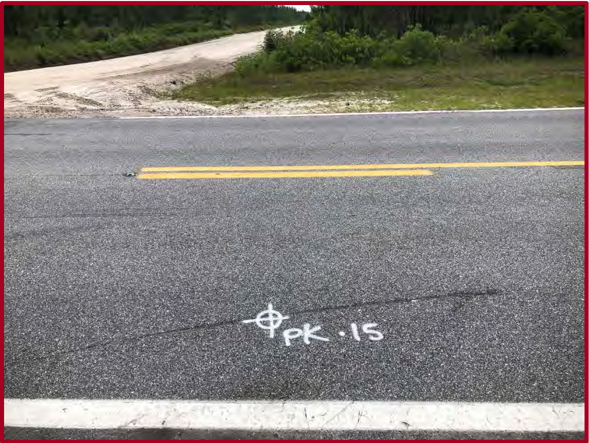
FIGURE D29: EXISTING CONDITIONS AT PAVEMENT CORE PK-15 (FACING WEST)
