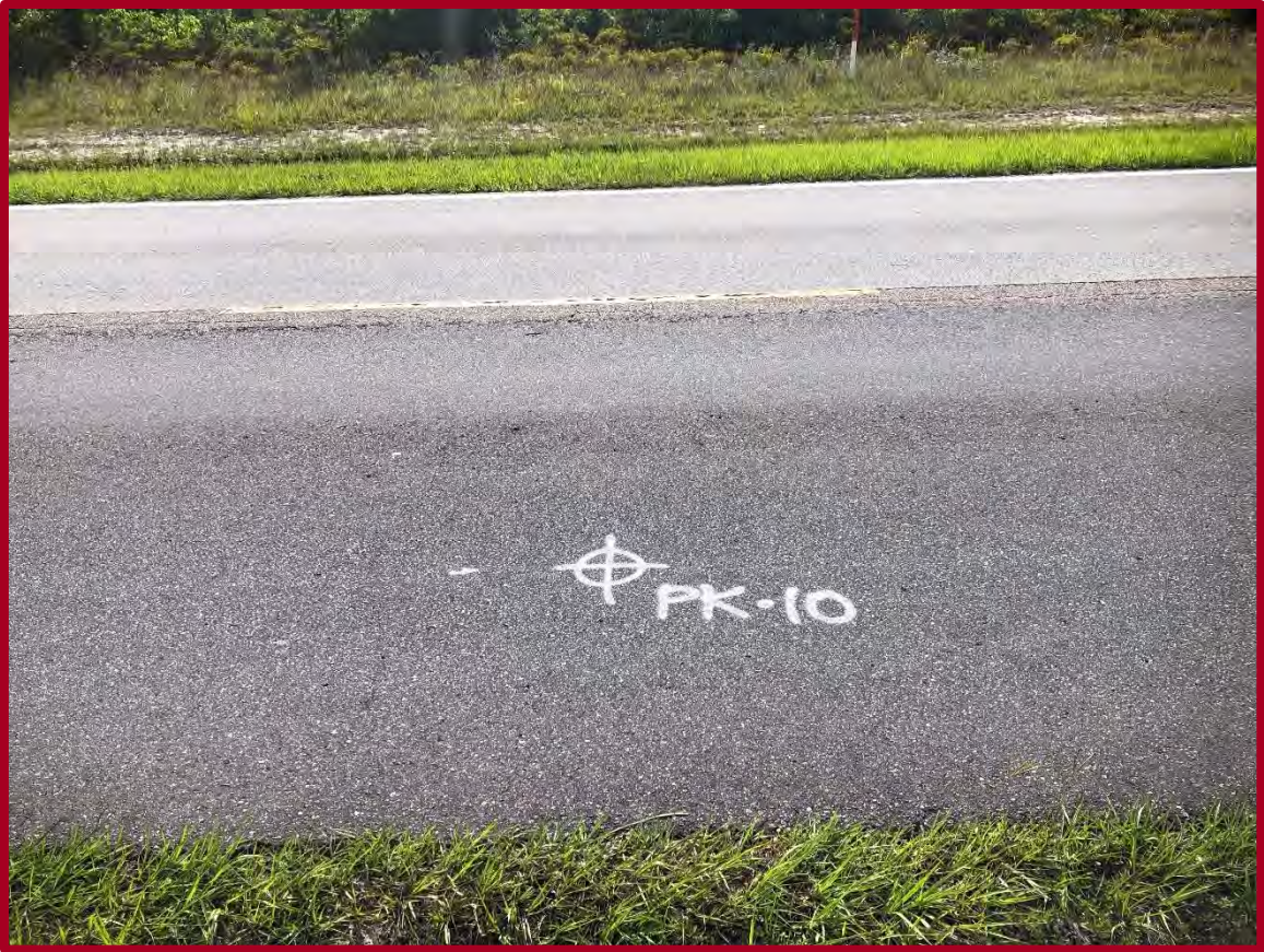
FIGURE D19: EXISTING CONDITIONS AT PAVEMENT CORE PK-10 (FACING EAST)
