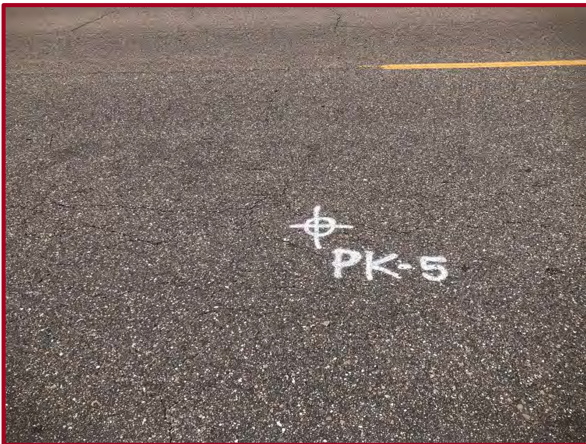
FIGURE D9: EXISTING CONDITIONS AT PAVEMENT CORE PK-5 (FACING WEST)
