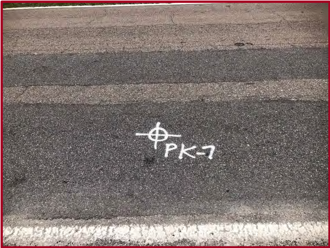
FIGURE D13: EXISTING CONDITIONS AT PAVEMENT CORE PK-7 (FACING WEST)
