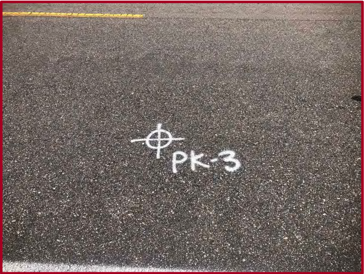
FIGURE D5: EXISTING CONDITIONS AT PAVEMENT CORE PK-3 (FACING WEST)
