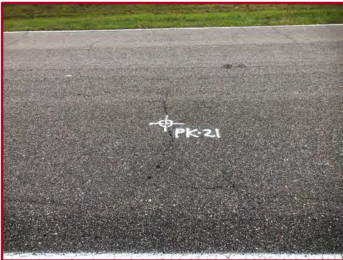
FIGURE D41: EXISTING CONDITIONS AT PAVEMENT CORE PK-21 (FACING WEST)
