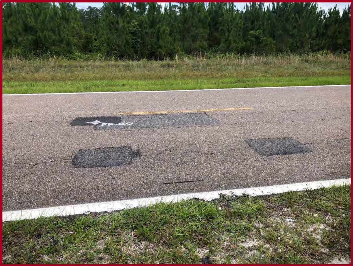
FIGURE D39: EXISTING CONDITIONS AT PAVEMENT CORE PK-20 (FACING EAST)
