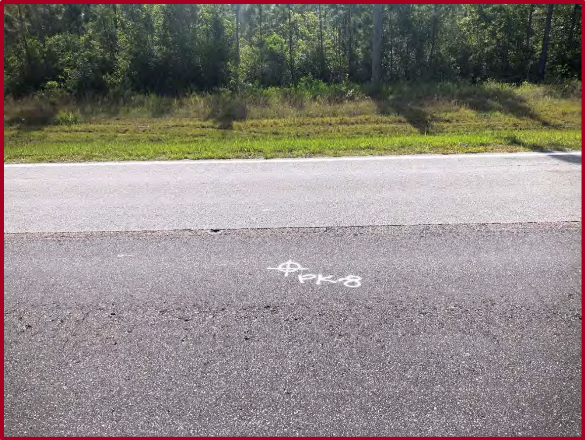
FIGURE D15: EXISTING CONDITIONS AT PAVEMENT CORE PK-8 (FACING EAST)
