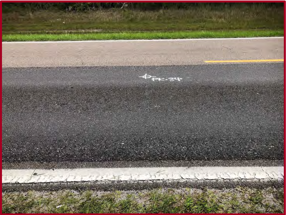
FIGURE D67: EXISTING CONDITIONS AT PAVEMENT CORE PK-34 (FACING EAST)
