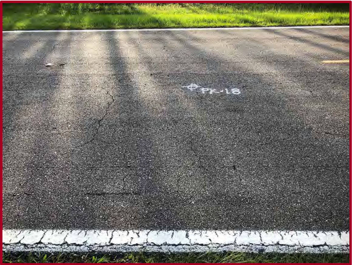
FIGURE D35: EXISTING CONDITIONS AT PAVEMENT CORE PK-18 (FACING EAST)
