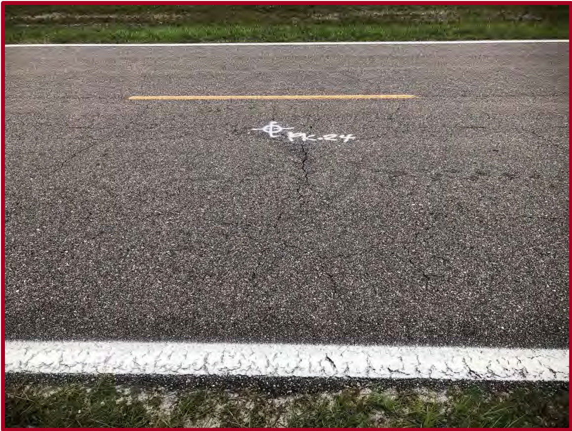
FIGURE D47: EXISTING CONDITIONS AT PAVEMENT CORE PK-24 (FACING EAST)
