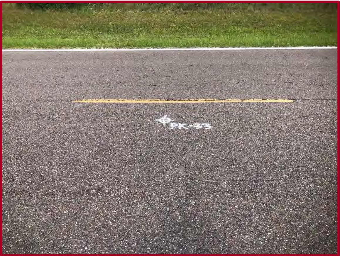
FIGURE D65: EXISTING CONDITIONS AT PAVEMENT CORE PK-33 (FACING WEST)
