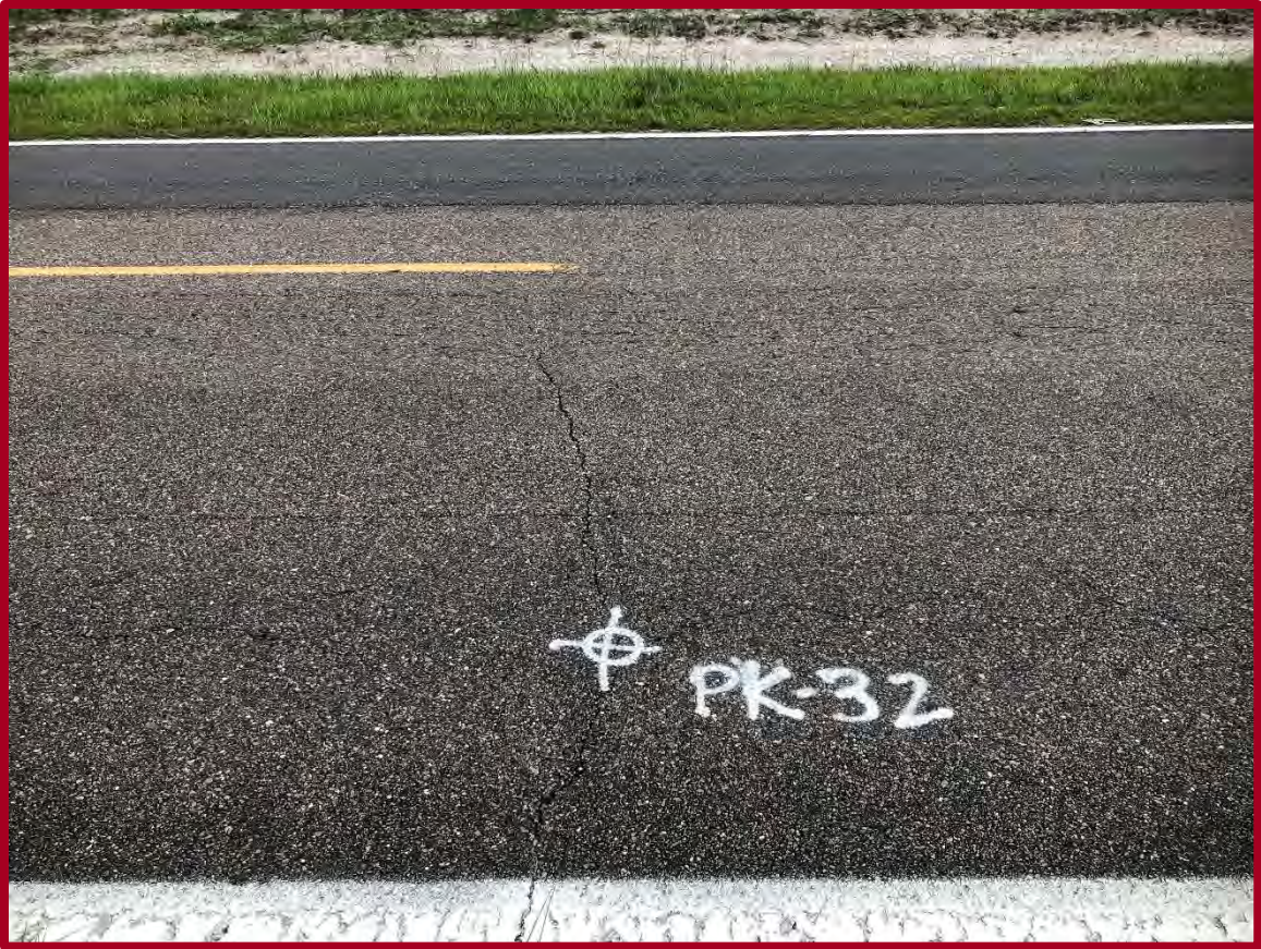
FIGURE D63: EXISTING CONDITIONS AT PAVEMENT CORE PK-32 (FACING EAST)
