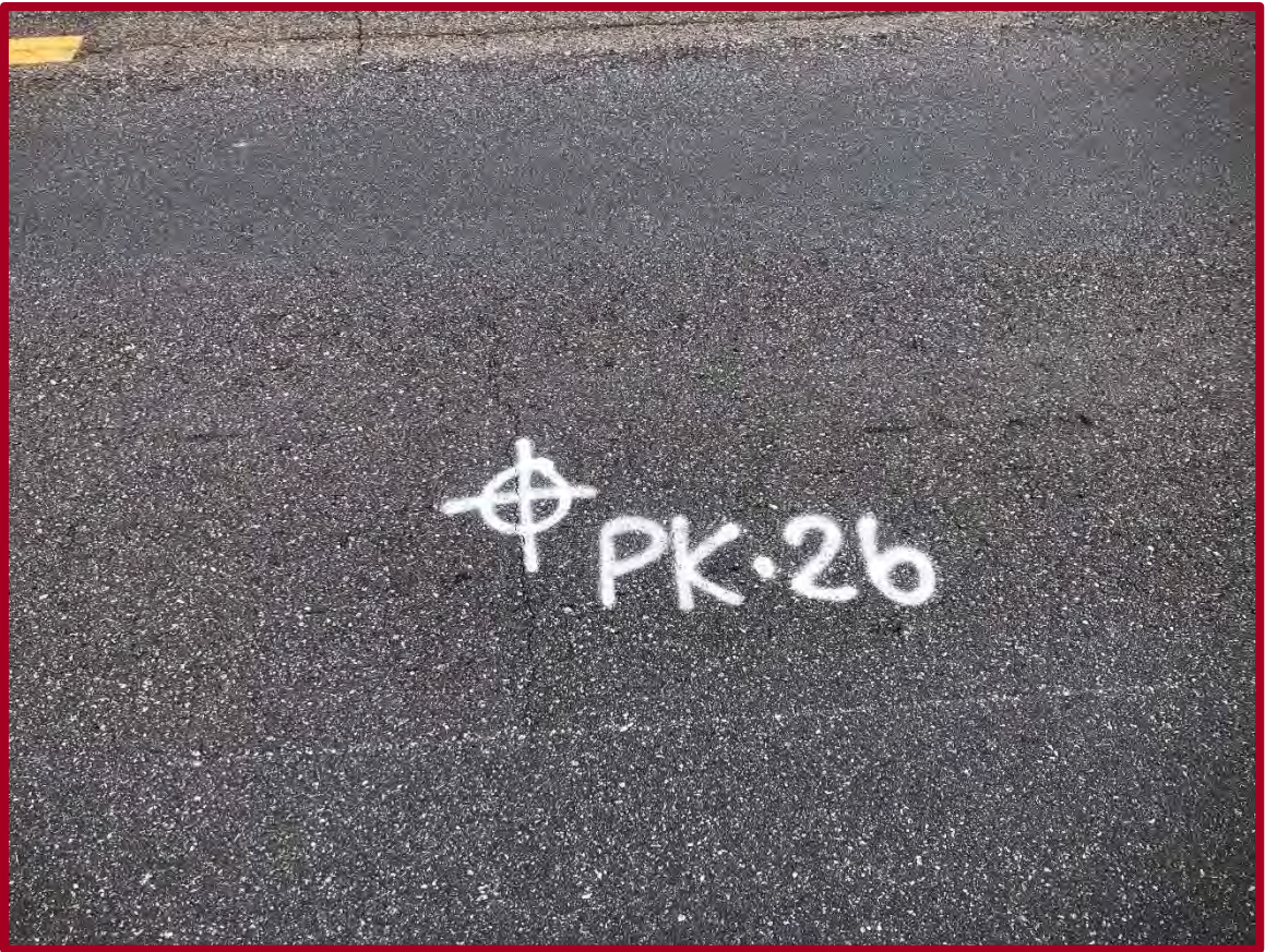
FIGURE D51: EXISTING CONDITIONS AT PAVEMENT CORE PK-26 (FACING EAST)
